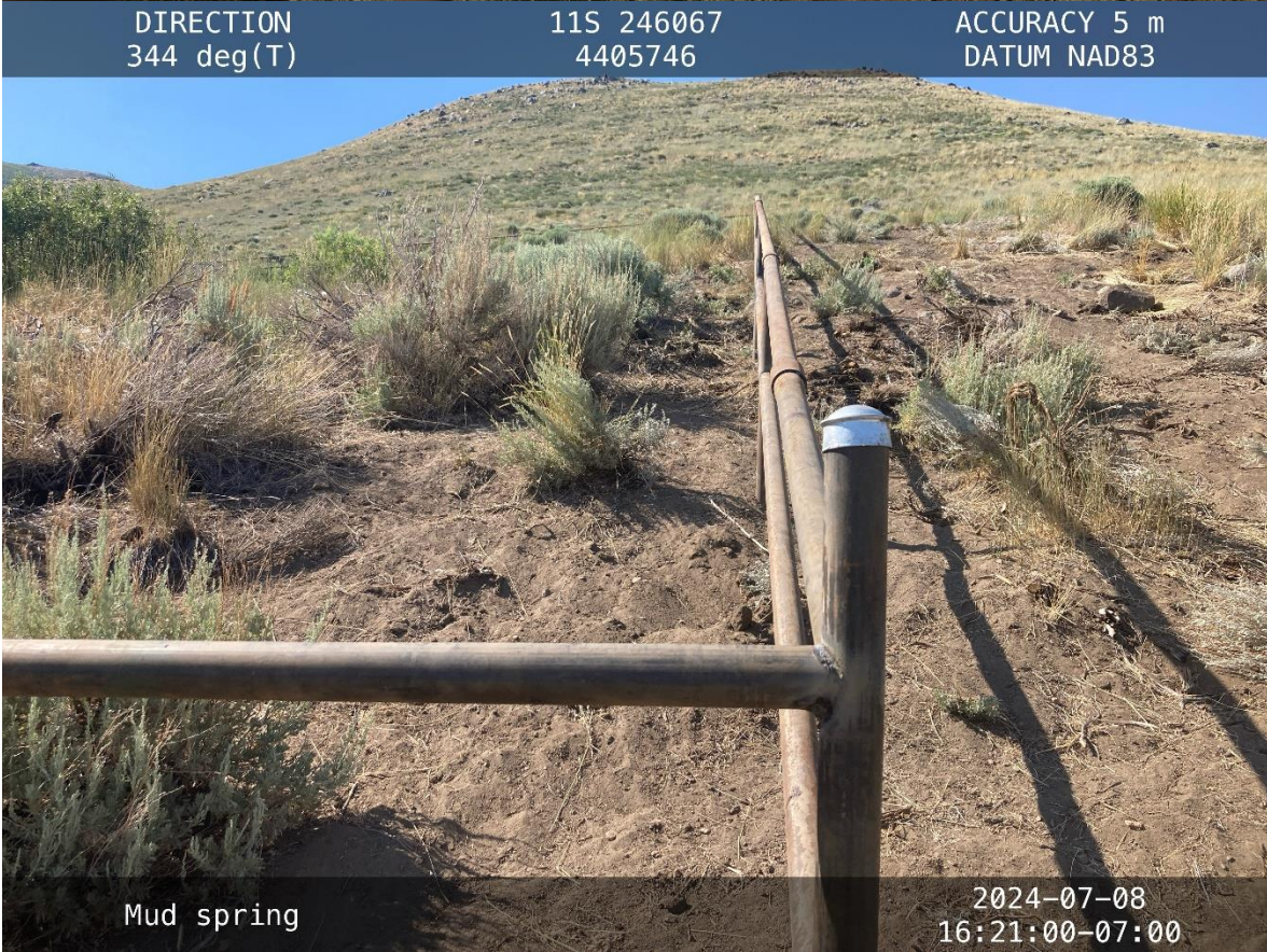
Figure 5. Photos of Mud spring with welded pipe rail fencing.
