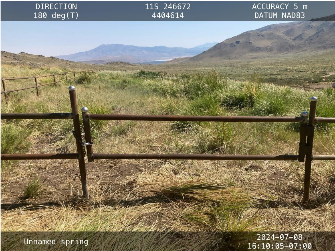
Figure 2. Photos of unnamed spring with welded pipe rail fencing.
